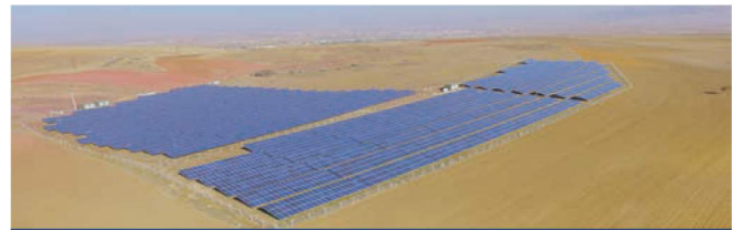
PHOTOVOLTAIC GROUND MOUNTED SPP 2017
