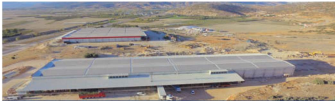
PHOTOVOLTAIC ROOFTOP MOUNTED SPP 2014
