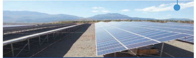
PHOTOVOLTAIC GROUND MOUNTED SPP 2016
