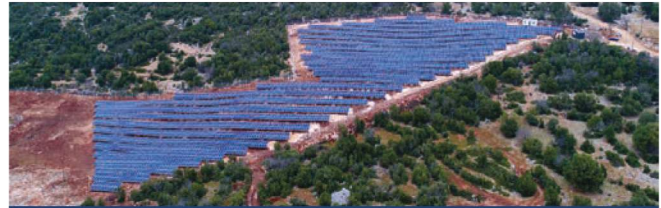
PHOTOVOLTAIC GROUND MOUNTED SPP 2017
