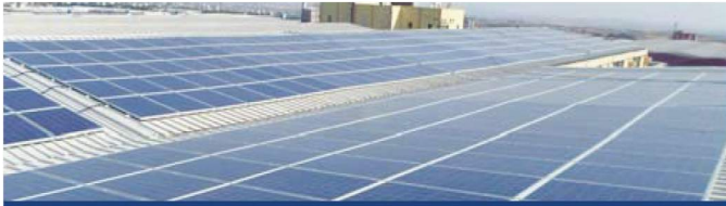
PHOTOVOLTAIC ROOFTOP MOUNTED SPP 2014
