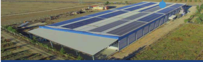
PHOTOVOLTAIC ROOFTOP MOUNTED SPP 2013
