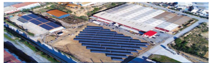
PHOTOVOLTAIC GROUND MOUNTED SPP 2017
