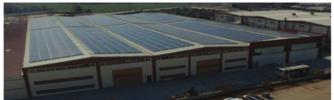
PHOTOVOLTAIC ROOFTOP MOUNTED SPP 2017
