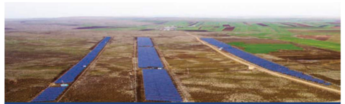
PHOTOVOLTAIC GROUND MOUNTED SPP 2015
