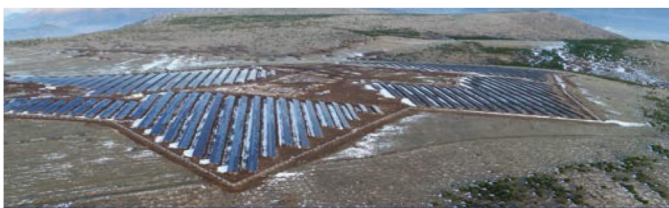
PHOTOVOLTAIC GROUND MOUNTED SPP 2017
