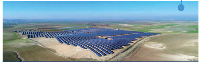
PHOTOVOLTAIC GROUND MOUNTED SPP 2017
