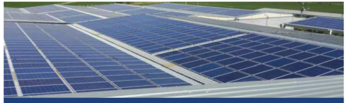
PHOTOVOLTAIC ROOFTOP MOUNTED SPP 2015
