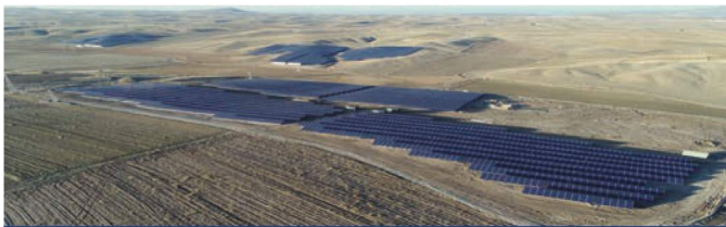
PHOTOVOLTAIC GROUND MOUNTED SPP 2017
