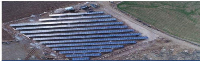
PHOTOVOLTAIC GROUND MOUNTED SPP 2017
