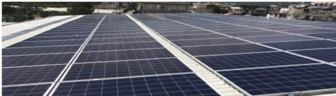
PHOTOVOLTAIC ROOFTOP MOUNTED SPP 2017
