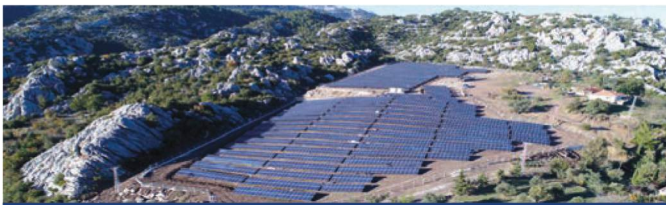
PHOTOVOLTAIC GROUND MOUNTED SPP 2017
