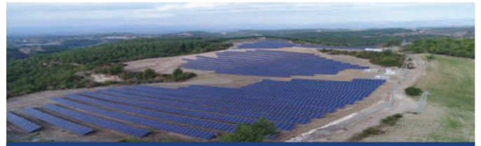
PHOTOVOLTAIC GROUND MOUNTED SPP 2017
