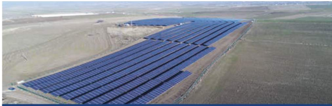
PHOTOVOLTAIC GROUND MOUNTED SPP 2017
