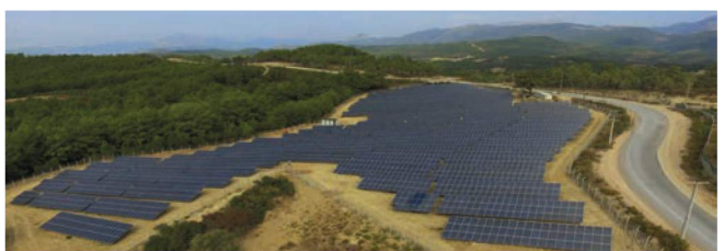
PHOTOVOLTAIC GROUND MOUNTED SPP 2016
