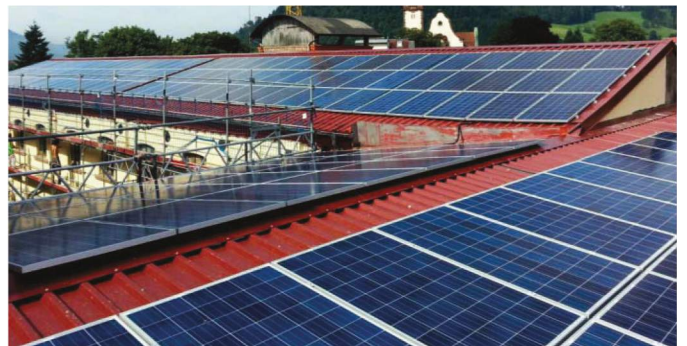
PHOTOVOLTAIC ROOFTOP MOUNTED SPP 2014
