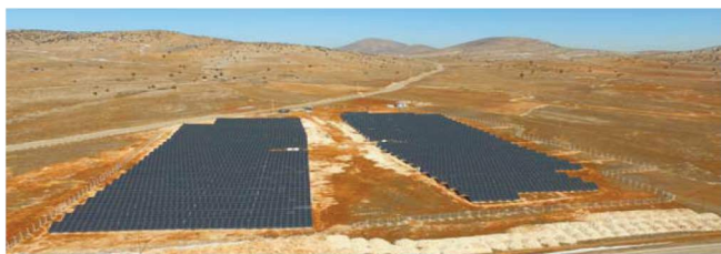
PHOTOVOLTAIC GROUND MOUNTED SPP 2016
