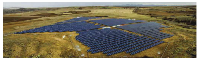
PHOTOVOLTAIC GROUND MOUNTED SPP 2016
