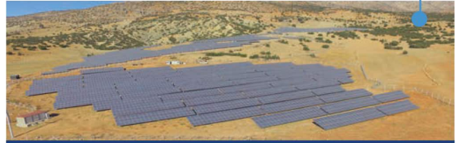
PHOTOVOLTAIC GROUND MOUNTED SPP 2016
