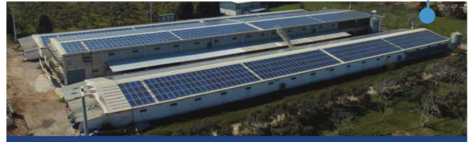
PHOTOVOLTAIC ROOFTOP MOUNTED SPP 2015
