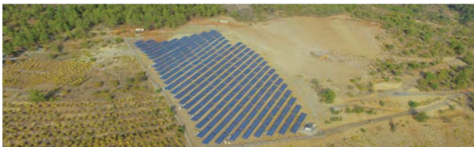
PHOTOVOLTAIC GROUND MOUNTED SPP 2016
