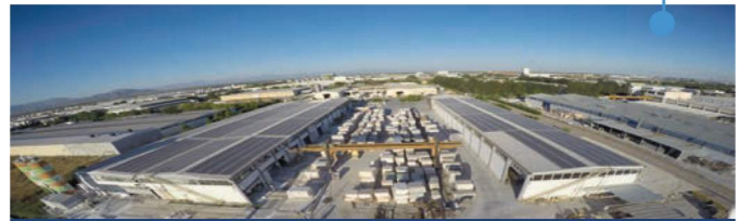
PHOTOVOLTAIC ROOFTOP MOUNTED SPP 2016
