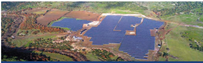
PHOTOVOLTAIC GROUND MOUNTED SPP 2017
