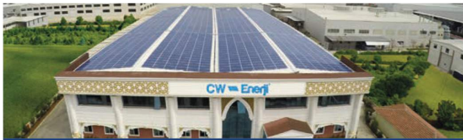
PHOTOVOLTAIC ROOFTOP MOUNTED SPP 2017
