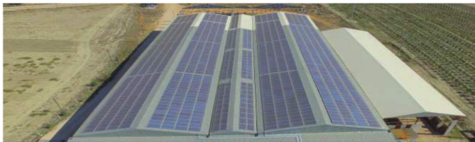
PHOTOVOLTAIC ROOFTOP MOUNTED SPP 2014
