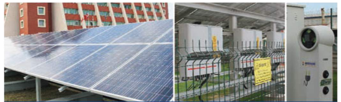
PHOTOVOLTAIC GROUND MOUNTED SPP 2014
