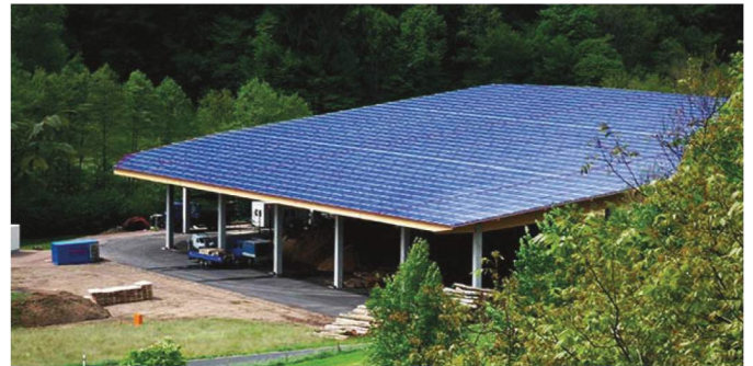
PHOTOVOLTAIC ROOFTOP MOUNTED SPP 2014
