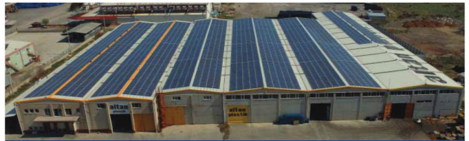
PHOTOVOLTAIC ROOFTOP MOUNTED SPP 2017
