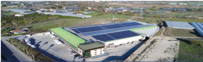
PHOTOVOLTAIC ROOFTOP MOUNTED SPP 2017
