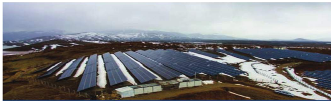
PHOTOVOLTAIC GROUND MOUNTED SPP 2015
