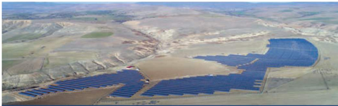
PHOTOVOLTAIC GROUND MOUNTED SPP 2017
