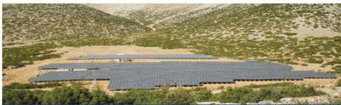
PHOTOVOLTAIC GROUND MOUNTED SPP 2016
