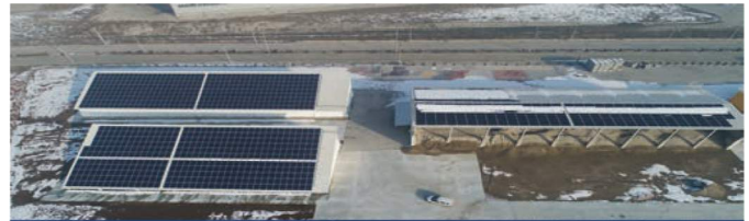
PHOTOVOLTAIC ROOFTOP MOUNTED SPP 2017
