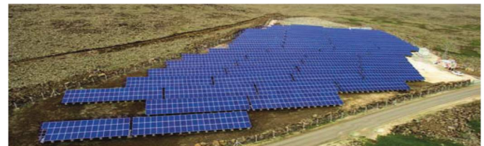
PHOTOVOLTAIC GROUND MOUNTED SPP 2017
