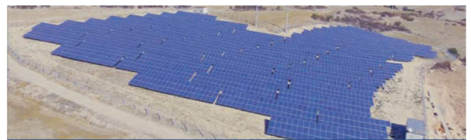
PHOTOVOLTAIC GROUND MOUNTED SPP 2015
