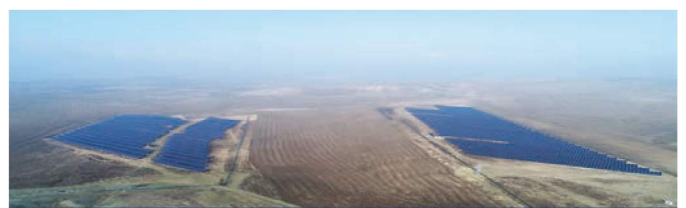
PHOTOVOLTAIC GROUND MOUNTED SPP 2017
