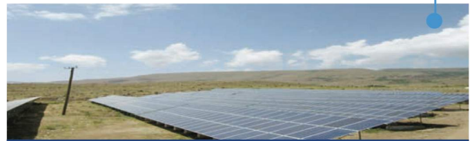
PHOTOVOLTAIC GROUND MOUNTED SPP 2017
