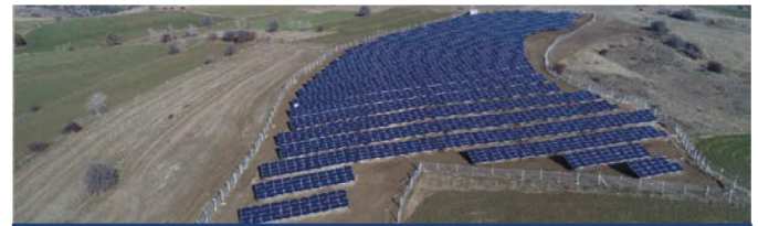
PHOTOVOLTAIC GROUND MOUNTED SPP 2017
