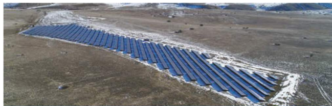
PHOTOVOLTAIC GROUND MOUNTED SPP 2017
