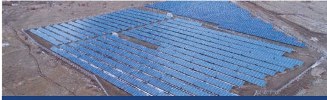
PHOTOVOLTAIC GROUND MOUNTED SPP 2017
