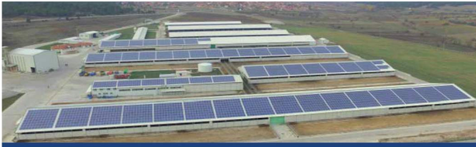
PHOTOVOLTAIC ROOFTOP MOUNTED SPP 2016
