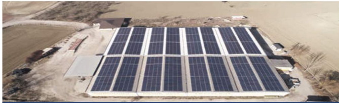
PHOTOVOLTAIC ROOFTOP MOUNTED SPP 2017
