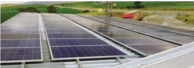
PHOTOVOLTAIC ROOFTOP MOUNTED SPP 2013
