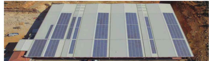
PHOTOVOLTAIC ROOFTOP MOUNTED SPP 2016
