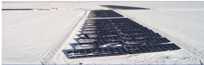
PHOTOVOLTAIC GROUND MOUNTED SPP 2017
