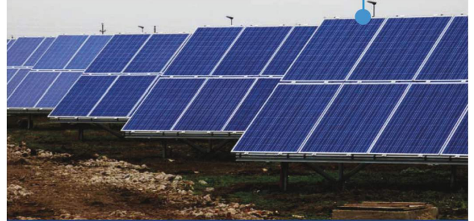
PHOTOVOLTAIC GROUND MOUNTED SPP 2014
