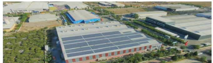
PHOTOVOLTAIC ROOFTOP MOUNTED SPP 2016
