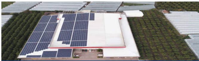
PHOTOVOLTAIC ROOFTOP MOUNTED SPP 2017
