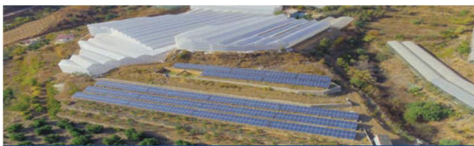
PHOTOVOLTAIC GROUND MOUNTED SPP 2013
